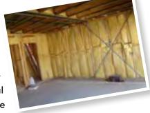
As there are many different kinds of insulation on the market (such as wool, fiberglass, and foam), the moisture risks for any given building's insulation can be difficult to predict. If moisture in a wall remains even after extensive removal efforts, contractors may have to open up the walls in order to test the moisture content of the insulation.
