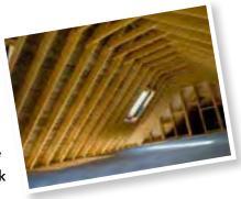
For the wood frame of the attic, either a pin-type meter or a pinless meter can be used to find moisture in the wood. In most cases, a pin meter can give you a more accurate reading of the depth of moisture penetration, while a pinless meter can allow you to scan more wooden beams more quickly.
