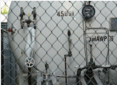
Difficult inspection sites
