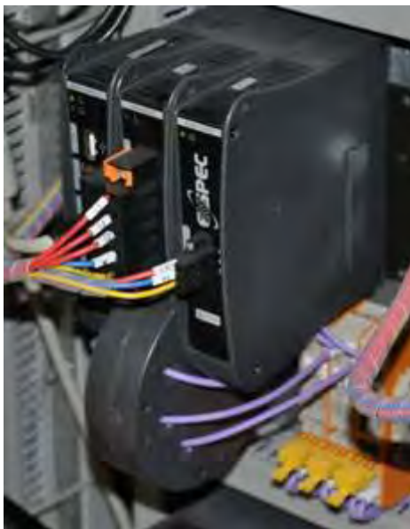
G4K Successful Current Wiring
