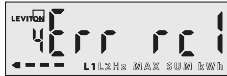
Error screen showing a reverse current installation error on Line 1
