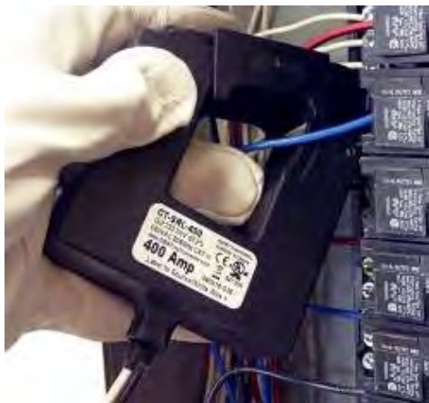
Photo 2: Install CT Around Conductor.
