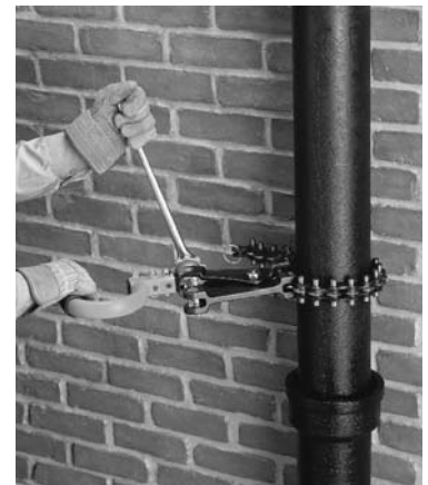
Cutting pipe in close quarters
