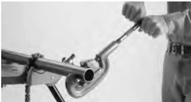
Figure 1 – Cutting End of Pipe
