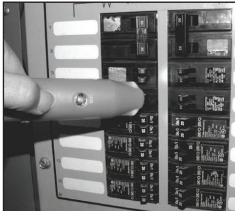
Identifying breaker by locating the "null".
