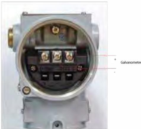
Test Terminal is marked as TEST on the terminal block. Connect TEST and negative terminal to the test terminal. Ensure that the voltage across the receptacles is kept below the diode threshold voltage so that no current passes through the diode. Make sure that the resistance of the test connection does not exceed 10 ohms while connecting an indicating meter or while taking the test readings. Note that a resistance of 30 ohms can cause an error of approximately 10% of actual value.
